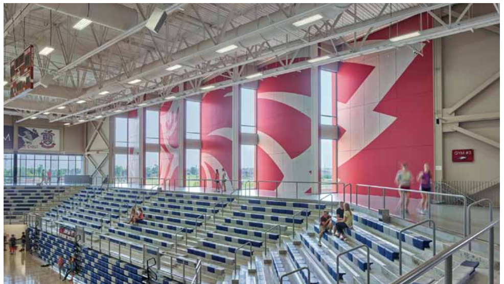
Joplin High School in Joplin, Mo., opened on Sept. 2, 2014. The new 488,000 square foot facility designed by DLR Group combines a college, career, and technology focused education along with Franklin Technology Center and a traditional high school campus. The facility has three state-of-the-art gymnasiums, including the Kaminsky Gymnasium pictured here. The Blueprint 220 team is looking at structures like this one at Joplin High School to get ideas for possible renovations in Barrington 220 School District.
