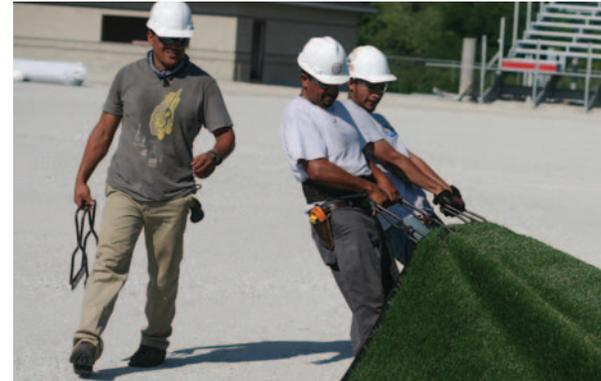
Workers unrolled sections of FieldTurf®, which were then sewn together and anchored to the playing surface of the new stadium.
