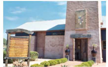
The entrance to Tower Estate in Hunter Valley, Australia. The brainchild of Len Evans, the estate includes a luxury hotel and conference center within its fortified Spanish hacienda-like walls.
